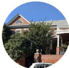
A Residential Unit at Bainbridge St
